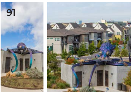
91 Park restrooms with sculpture
