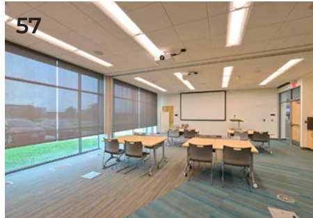
57 Motorized window shades to control sunlight
