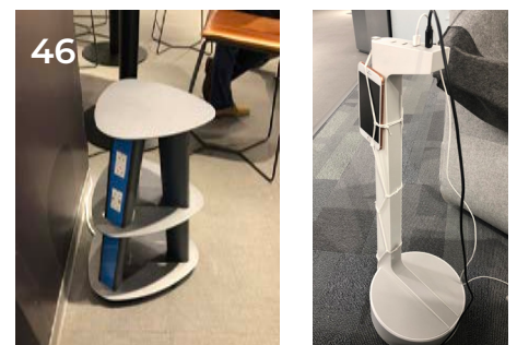
46 Mobile power towers to provide additional outlets throughout the space as needed
